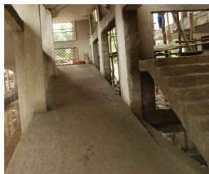
New structure funded by WB with appropriate ramp
